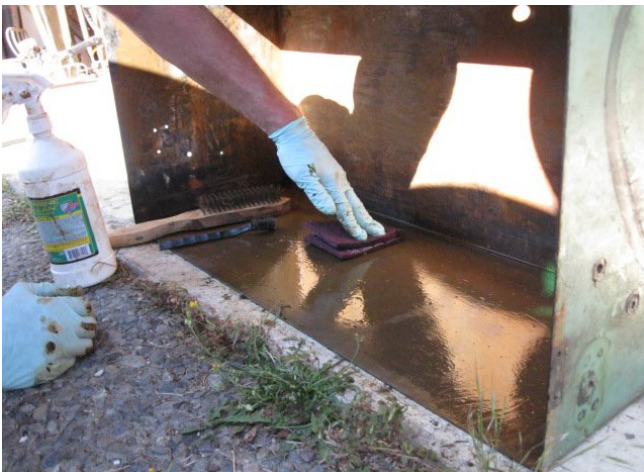
Using POR 15 degreaser, wire brushes, and red Scotch-Brite
