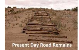
California State Highway Commission took authority for the road and upgraded the route to an 8-foot wide wood roadbed. Turnouts were added about a mile apart in order to let the traffic flow in both directions. When sand covered the road, a horse team was brought in and the sections were lifted and dusted off and laid back down and traffic resumed. Portions of the plank road were moved by teams of mules when the shifting sand made such corrections necessary.
